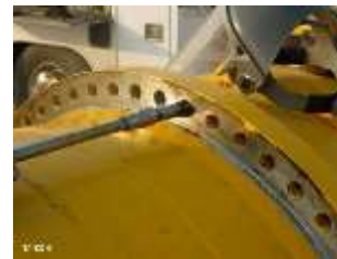
Cleaning paint and rust prior to torquing
